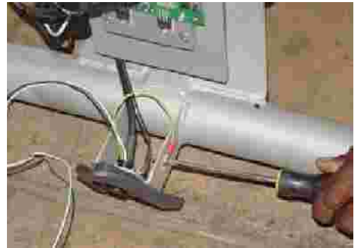
Figure 18 - Remove ground wire screw
